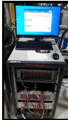
SM18 superconducting magnet test stands
